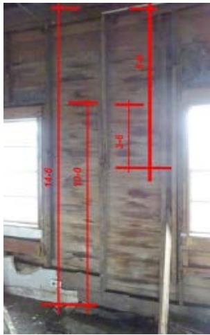
Figure 10. Phase 1 Walls, 8 and 10 Foot Stud "Sistered" to Make a 14'-6 Stud Height Source: Michael O'Brien Image.
