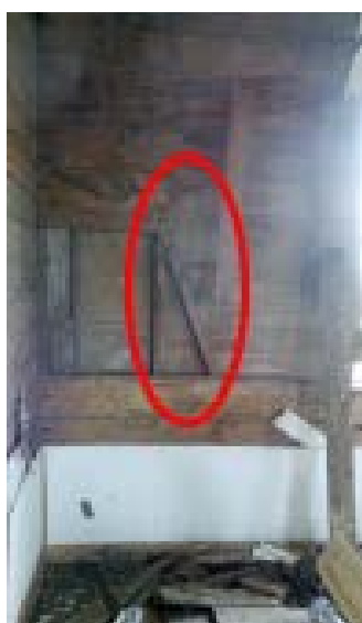
Figure 9. Downbrace (Circled) in Southeast Corner at South Tower Door
