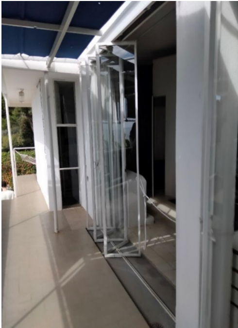
Figure 2. Villa E.1027, fenêtres en longueur . “...Not only does each room have its own balcony with access to the outside, but the fixtures, shutters, windows are all removable...”
