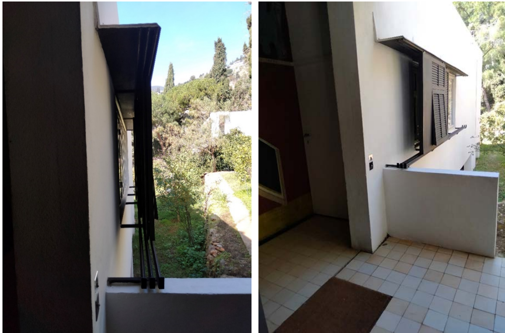
Figure 3. Villa E.1027, details. “...a vernacular Niçoise shutter adapted to the strip window enabled the occupant to manipulate outward views and penetration of the sun's rays, admitting natural ventilation while protecting internal privacy...” Source: Pittaluga 2023.
