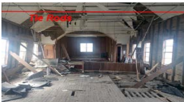
Figure 13. Interior Demolition 28 Jan. 2017 Showing Tie Rods, Semi-Cathedral Ceiling
