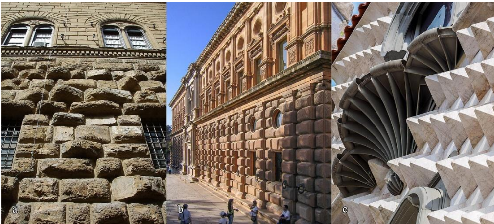
Figure 3. Different typologies of rustication: a) the façade of the Medici-Riccardi palace in Florence (1444-1484, Italy); b) the southern façade of the Palace of Charles V in Granada (1527-1623, Spain); a detail of the House of the Beaks in Lisbon (Portugal, 1523)
