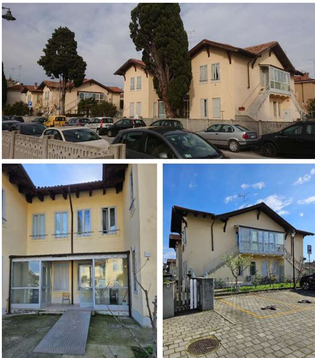
Figure 8. Views of the 'H-type' Housing in the Workers' Village of Panzano (Recent additions are visible on the ground floor and above the balcony, protecting entrances to dwellings)
