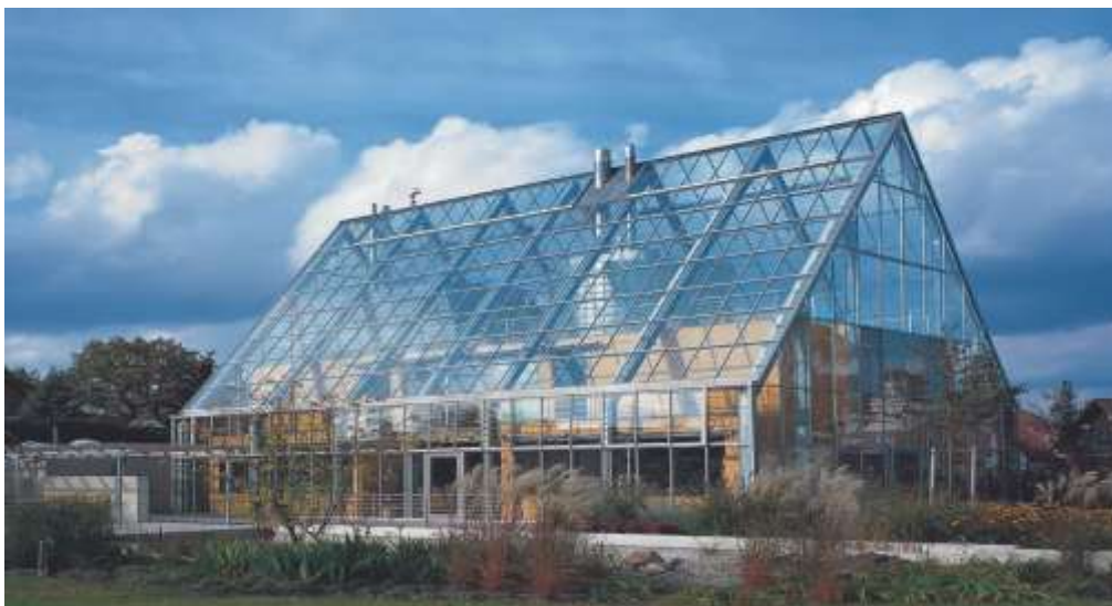
Figure 4. Niederwöhrmeier + Kief's residential project in Nuremberg (2000) (The greenhouse envelope becomes the primary architectural element that encapsulates and protects the dwelling within)
