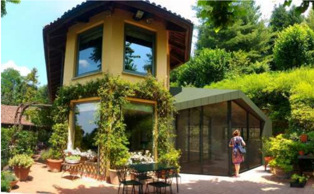
Figure 2. ACC Naturale Architettura Cristiana Catino, in Superga, Turin (The greenhouse operates as an environmental mediator that harmonizes with both existing architecture and landscape context)
