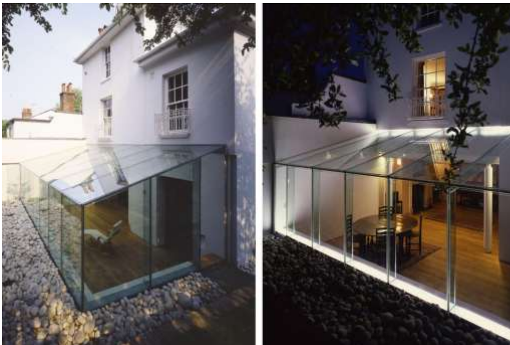
Figure 1. Architect Rick Mather's Glass Addition to a Georgian Cottage in Hampstead, London (1991/1992), North Facing Elevation (A Transparent addition that extends the living space while maintaining a clear distinction between the original building and the new intervention)
