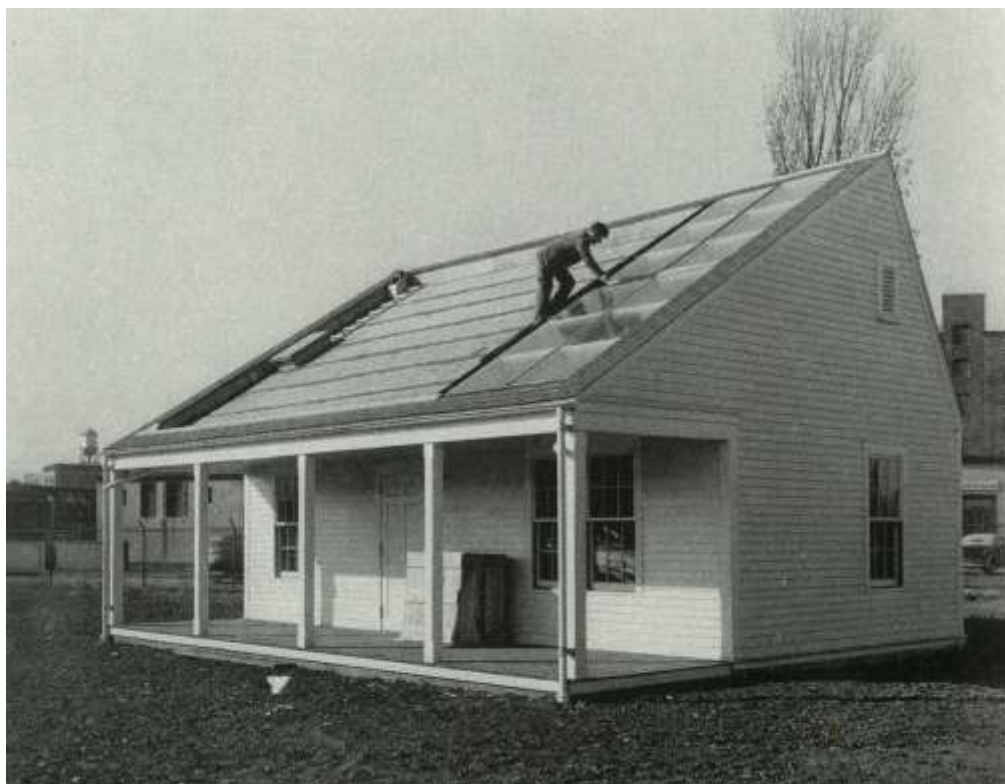
Figure 2. MIT Solar House I, Cambridge, Massachusetts, 1939. Installation of ‘Solar Collectors’ on the Roof of the First ‘Solar House’ Prototype, developed by the Research Group Led by Hoyt Clarke Hottel on the Campus of the Massachusetts Institute of Technology (MIT)
