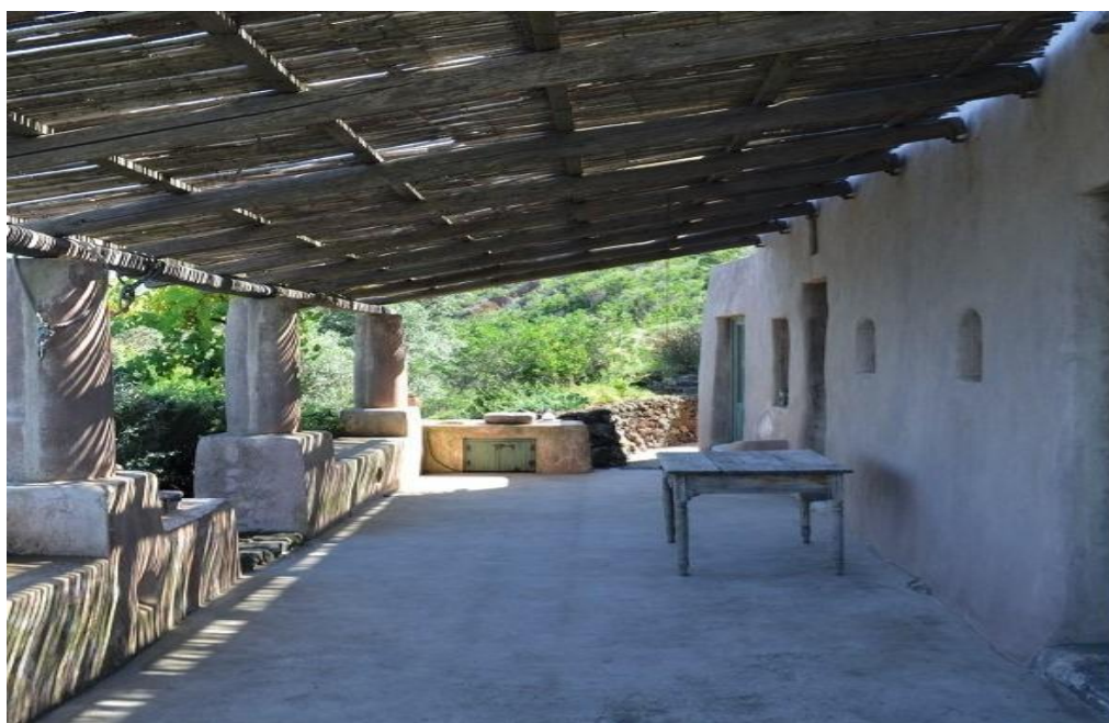
Figure 5. A Typical Aeolian House: We Can See the Bagghiu and its Pergola in Reed Mat
