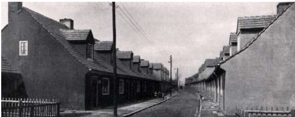
Figure 8. Paul Schreiber, Small Houses Estate, Tarnogaj, Kamieniecka Street, 1920
