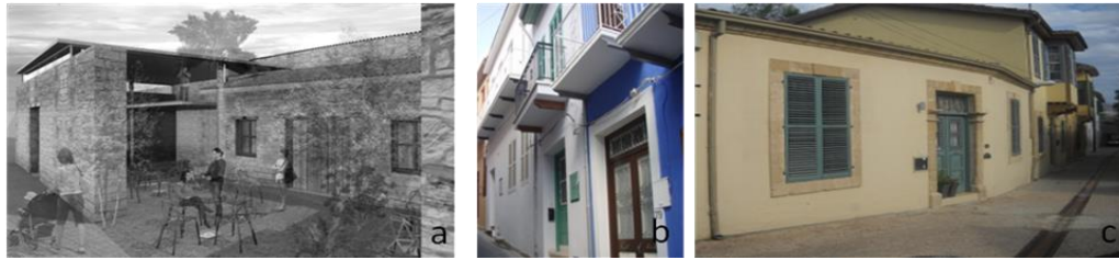
Figure 5. Different Strategies for Completing the Form of Traditional Dwellings a: with the Use of New Materials and Style, b,c: without any Distinction between the Old and New
