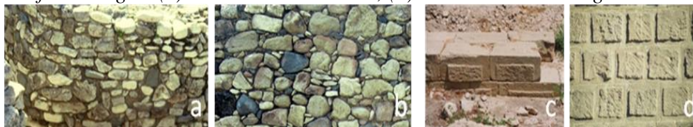
Figure 2. Different Types of Stone Walls. Walls with Rubble Stones (a) Prehistoric Structure, (b) Traditional Dwelling and Walls with Ashlar Showing Drafted Margins (c) Prehistoric Structure, (d) Traditional Building
