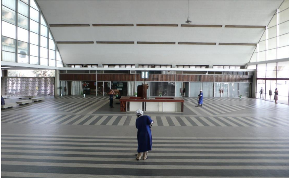
Figures 16. Beira Railway Station, Beira, Mozambique (1958-1966). João Garizo do Carmo, Paulo Melo Sampaio, Francisco José de Castro Source: Ana Magalhães, 2008.
