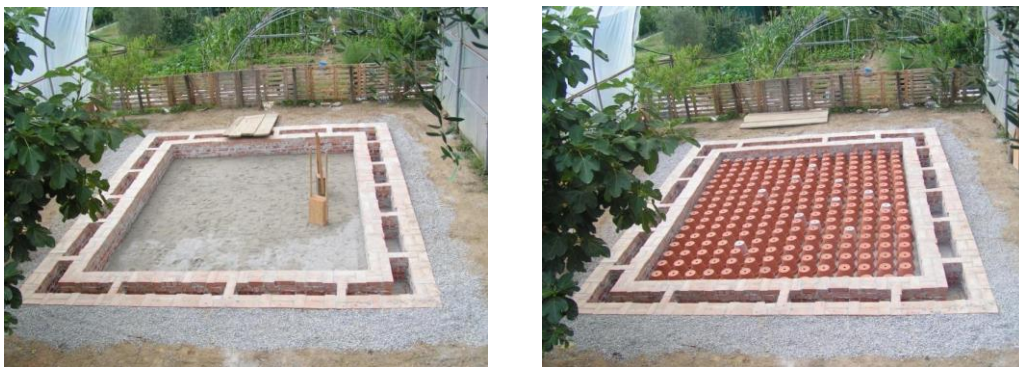
Figure 4. Straw-bale Construction in Sestri Levante (Genoa), Foundation (left), Hornet's Nest (right)
