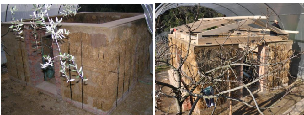
Figure 5. Straw-bale Construction in Sestri Levante (Genoa), Masonry (left), Roof (right)
