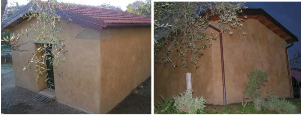
Figure 6. Straw-bale Construction in Sestri Levante (Genoa)
