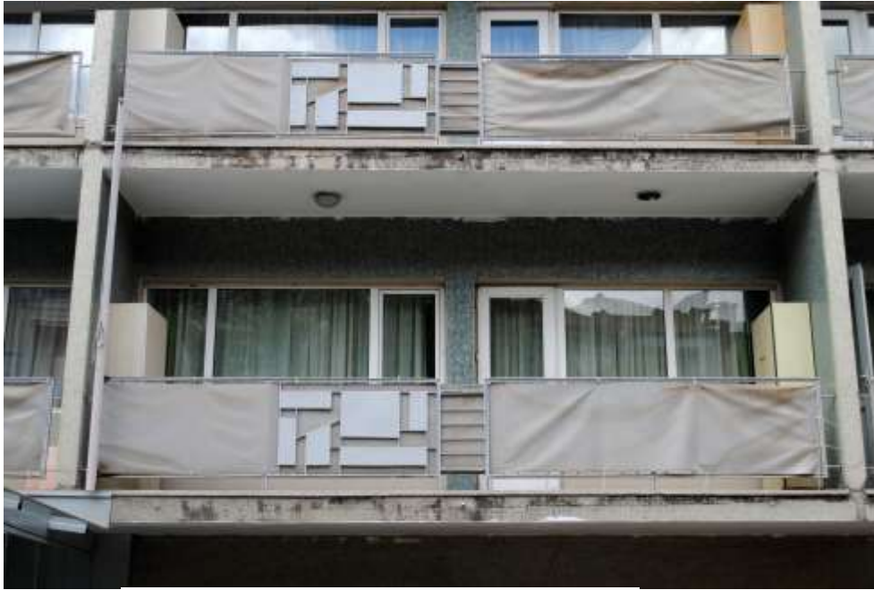
Figure 4. Ankara Balcony Railings, District 2 (Kızılay) Source: The author's archive.
