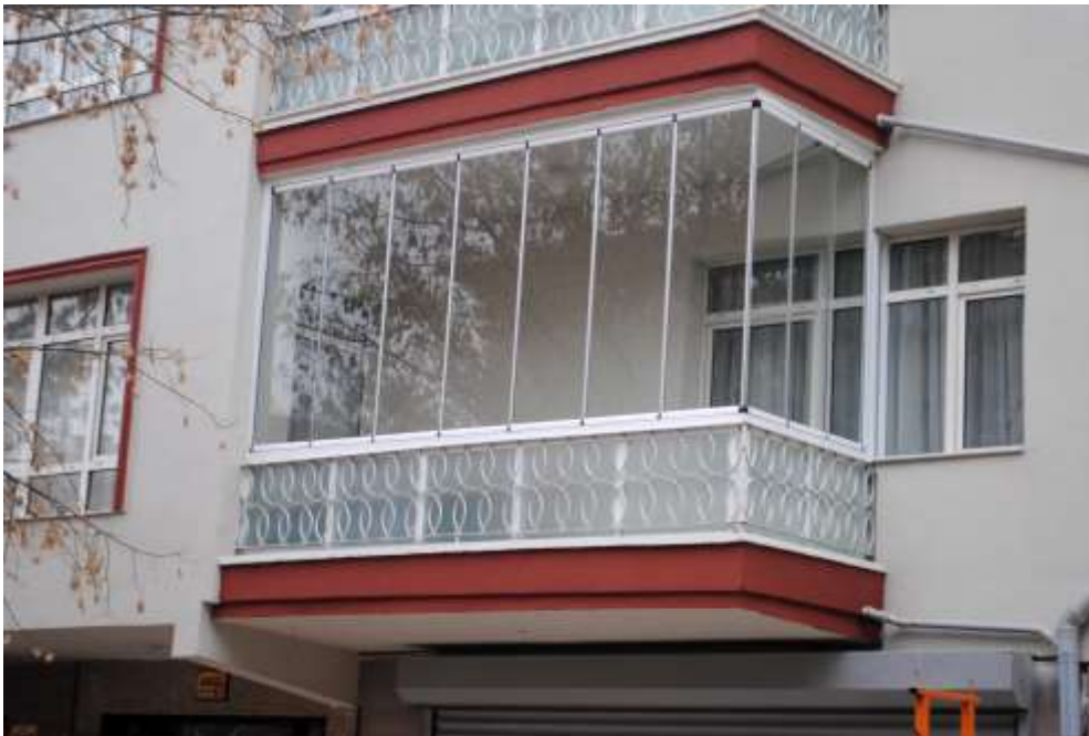
Figure 7. Ankara Balcony Railings, District 5 (Anittepe)
