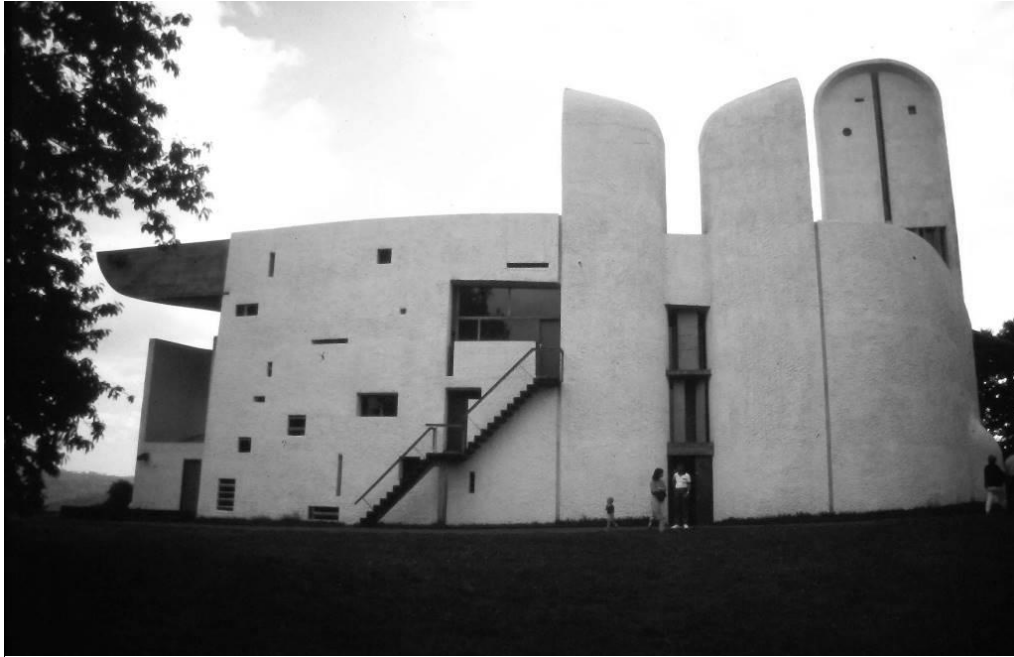
Figure 6. Exterior View of Notre-Dame-du-Haut (1950-55) in Ronchamp, France. Le Corbusier Source: Author, 1991.
