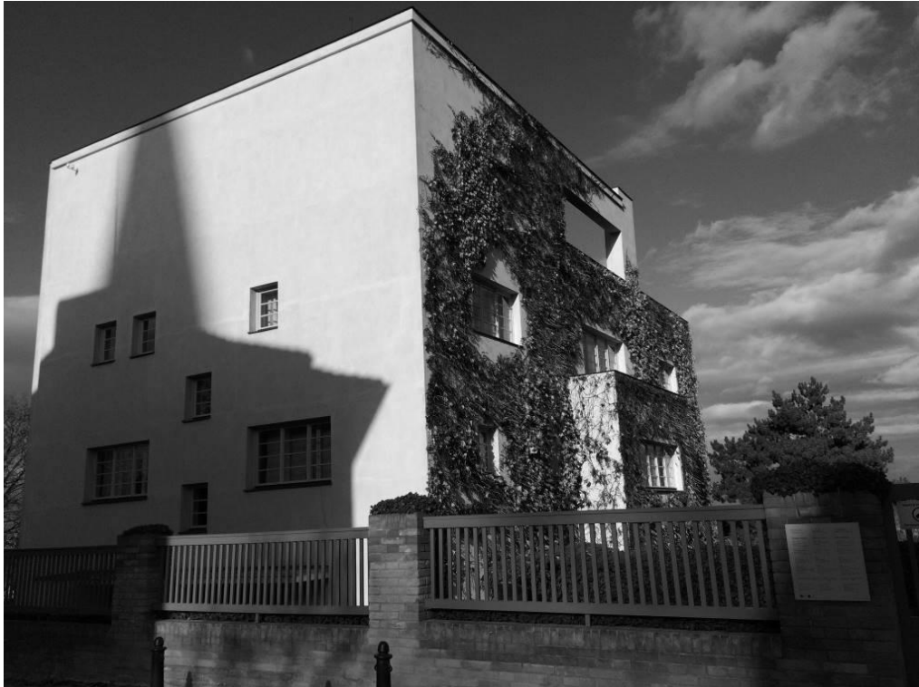
Figure 2. Exterior View of Villa Müller (1928-30) in Prague, Czech Republic. Adolf Loos
