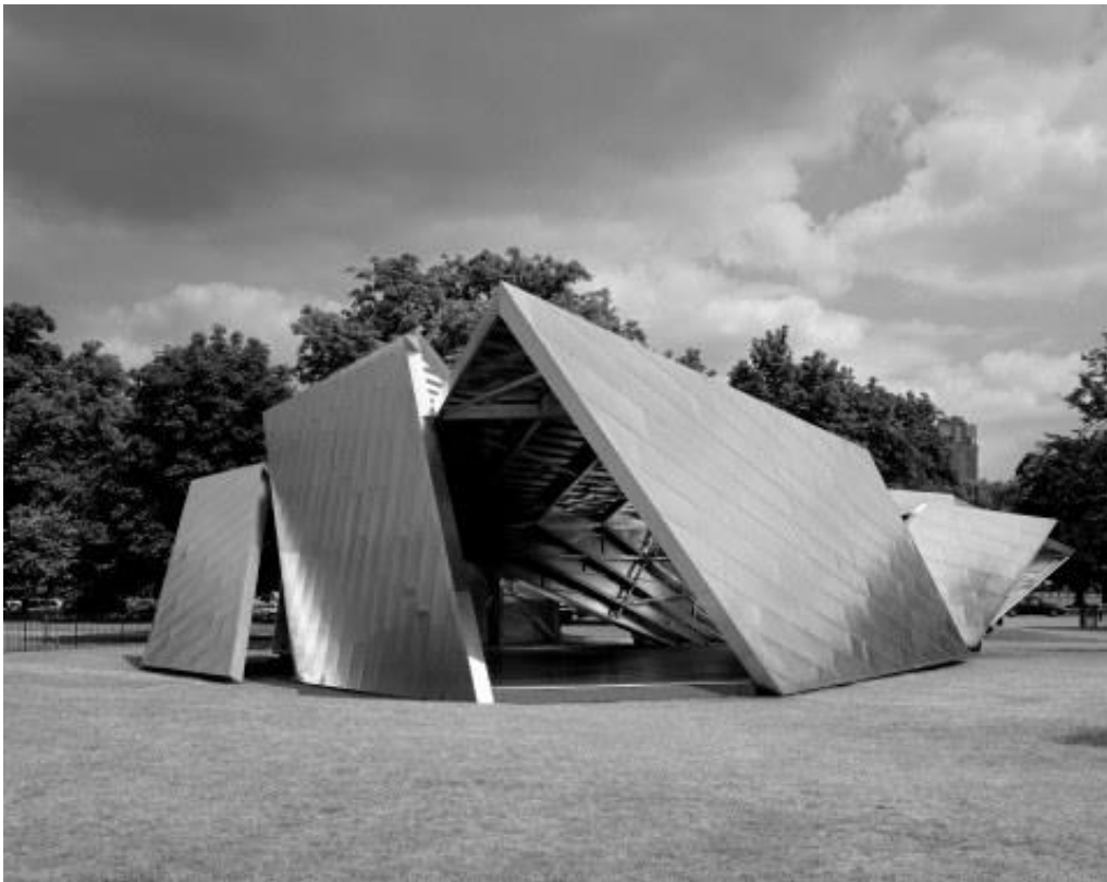
Figure 2. The 2001 Serpentine Gallery Pavilion by Daniel Libeskind Source: Serpentine Gallery 5 May 2018. www.serpentinegallery.org .
