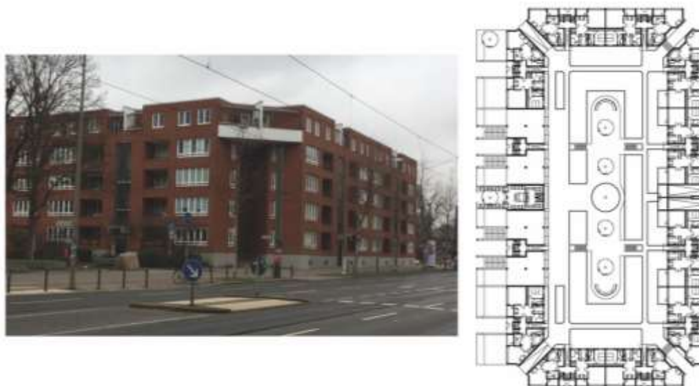
Figure 5. Block 270 on Vinetaplatz. View from the Street and Ground Floor Plan Source: Left: Photo by the author (2018). Right: © Kleihues+Kleihues.
