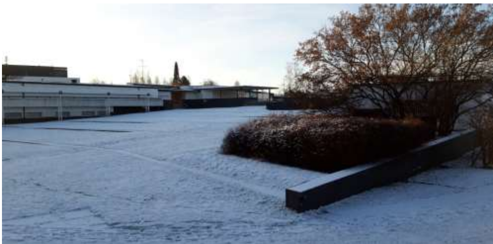
Figure 2. Seinäjoki Parish Centre Seen from the Church Yard
