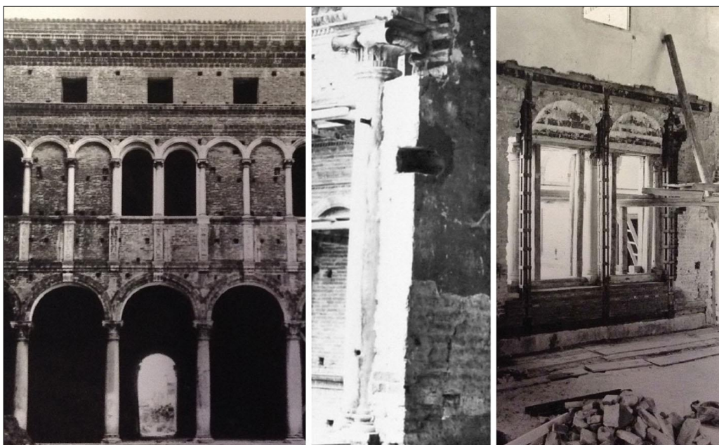
Figure 19. Historical Photographs before the Restorations; the Third Image Shows the Moment when the Restorations Destroyed the Walls behind the Columns Source: Images Preserved in the Archive of the Ministry of Culture in Ravenna.
