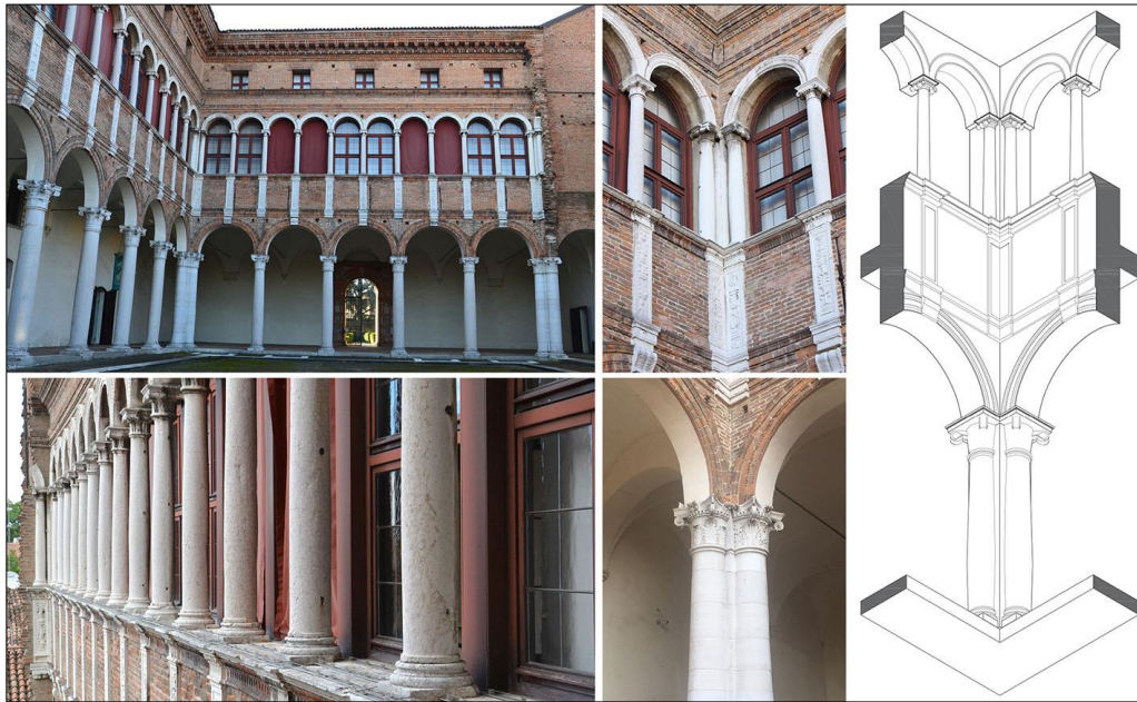
Figure 14. On the Left, Images of the Courtyard and, on the Right, an Axonometric Drawing of the Corner Solution
