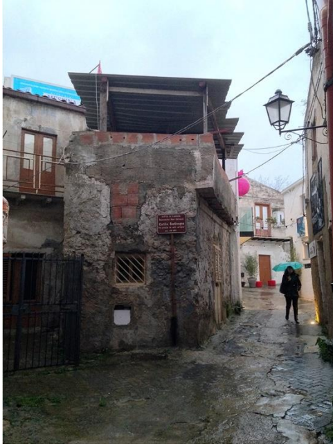
Figure 1. Cortile Bentivegna before Farm's Project Source: Di Carlentini and Liotta. 65
