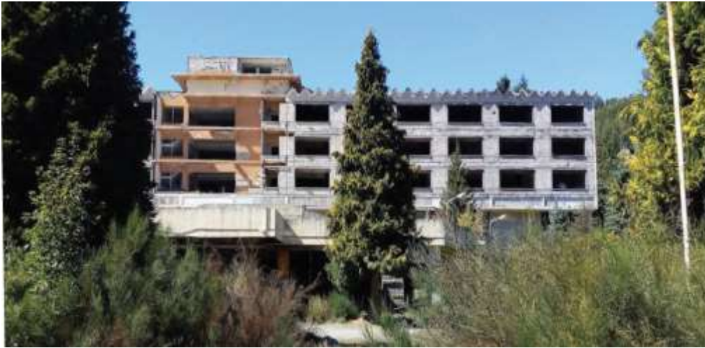
Figure 4. Current State of the Building (Photo by Authors)
