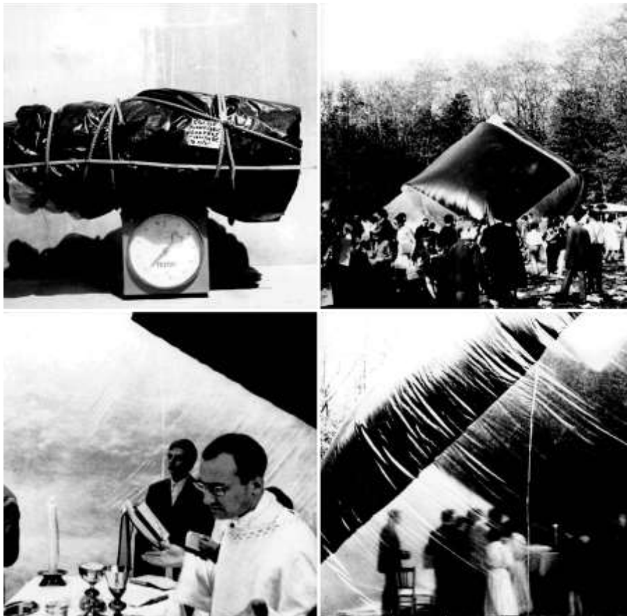
Figure 6. Ephemeral Church, Hans Walter Müller. The Chapel Folded, During the Inflation Process and in Use
