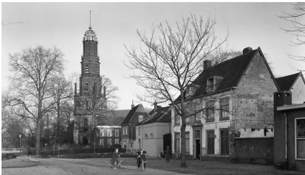
Figure 2. IJsselstein, the Renaissance Tower of the Dutch Reformed or Old Saint Nicholas Church, Designed by A. Pasqualini (1532-35) with Expressionist Spire by Michel de Klerk as Post-Fire Restoration (1921-23) in 1962
