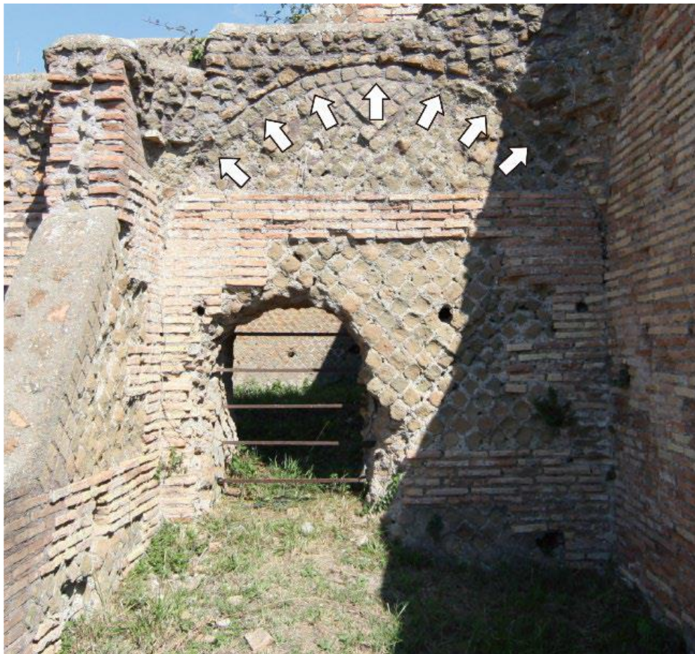
Figure 3. Outling Lunet Seen in Opus Reticulatum
