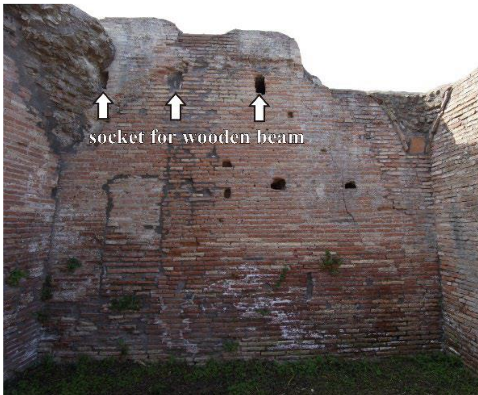
Figure 6. Conversion from Wooden-Beam-support to Cross-Vault-Support
