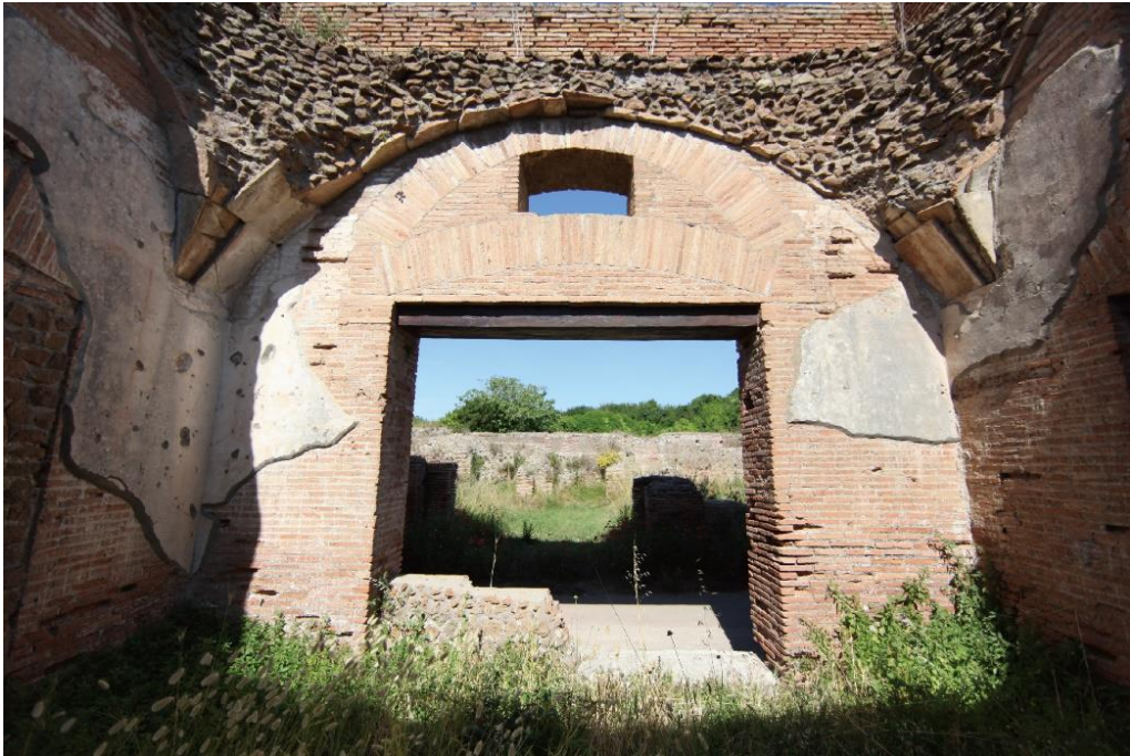
Figure 2. Example of Collapsed Cross Vault (House of Annius)
