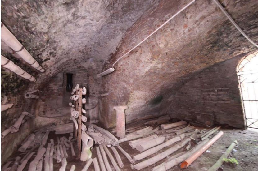
Figure 11. Barrel vaults of Capitolium
