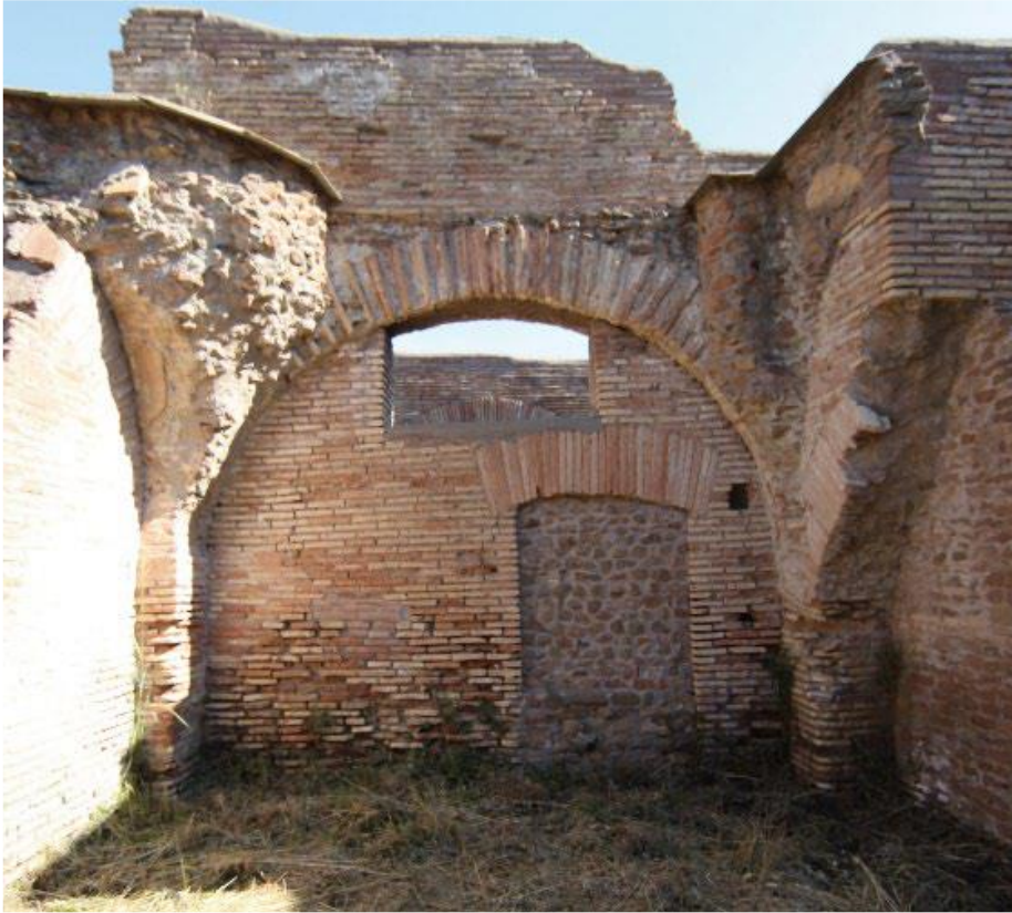
Figure 5. Building Partition Wall under Cross Vault
