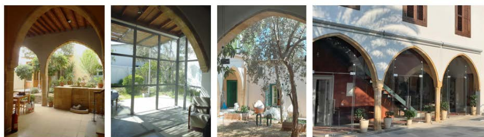
Figure 11. Semi-Open Spaces Preserved in Their Original Character (Left) or Converted into Closed Areas with the Use of Glass Surfaces (Three Examples to the Right)
