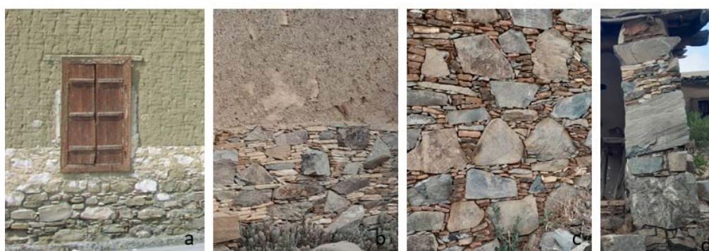
Figure 13. Traditional Masonries (Stone, Adobes) in Rural Settlements
