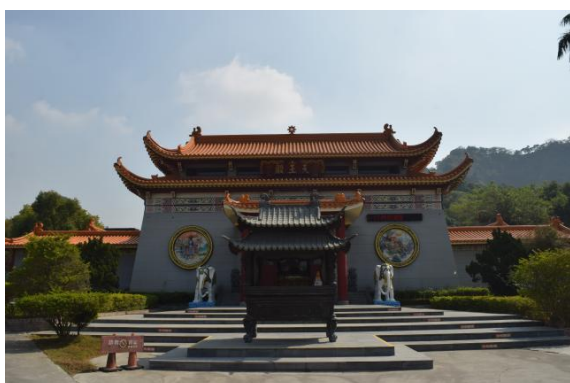
Figure 17. The Exterior of the Hall of Heavenly Kings, with the Northern Roof
