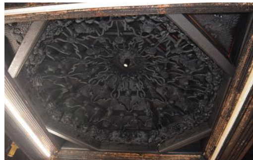
Figure 26. Octagonal Wood Carving Ceiling
