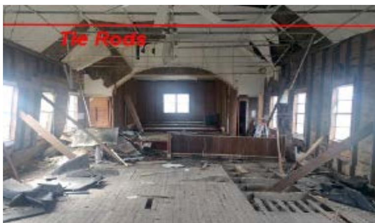
Figure 13. Interior Demolition 28 Jan. 2017 Showing Tie Rods, Semi-Cathedral Ceiling
