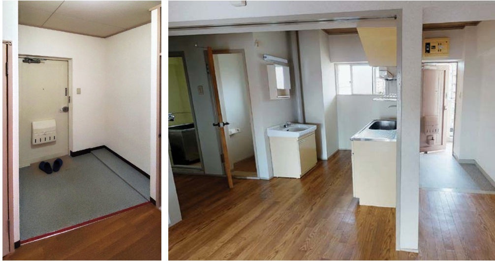
Figure 23. Examples of the Entrance Space in Nagoya Municipal Housing Source: authors.
