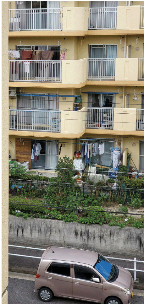
Figure 27. Example of Balconies in Nagoya Municipal Housing Units which also Play the Role of Evacuation Route in Case of Disaster Source: authors.
