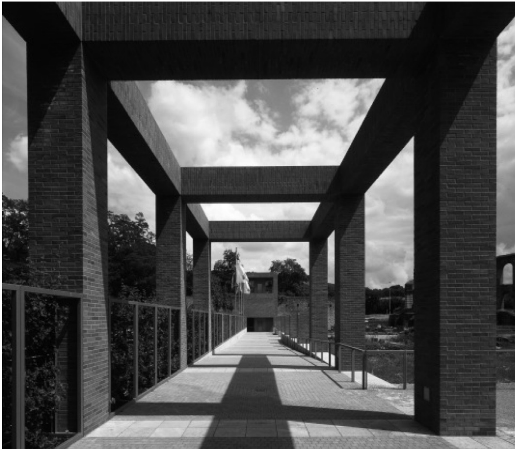
Figure 10. Entrance to the Kaiserthermen
