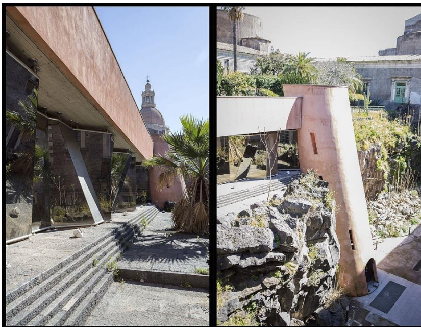
Figure 4. Recovery of the Compleso dei Benedettini, Catania, Giancarlo De Carlo (1986-2004). On the left: the glass wall of the new thermal power plant under the Giardino dei Novizi, where the Monastery is narrated through fragments and broken images that reflect along a sequence of rectangles with different inclinations. On the right: the helical staircase, nestled between the lava rock and the floor level of the Giardino dei Novizi, concludes the sequence of overlapping "interrupted signs," both natural and man-made.
