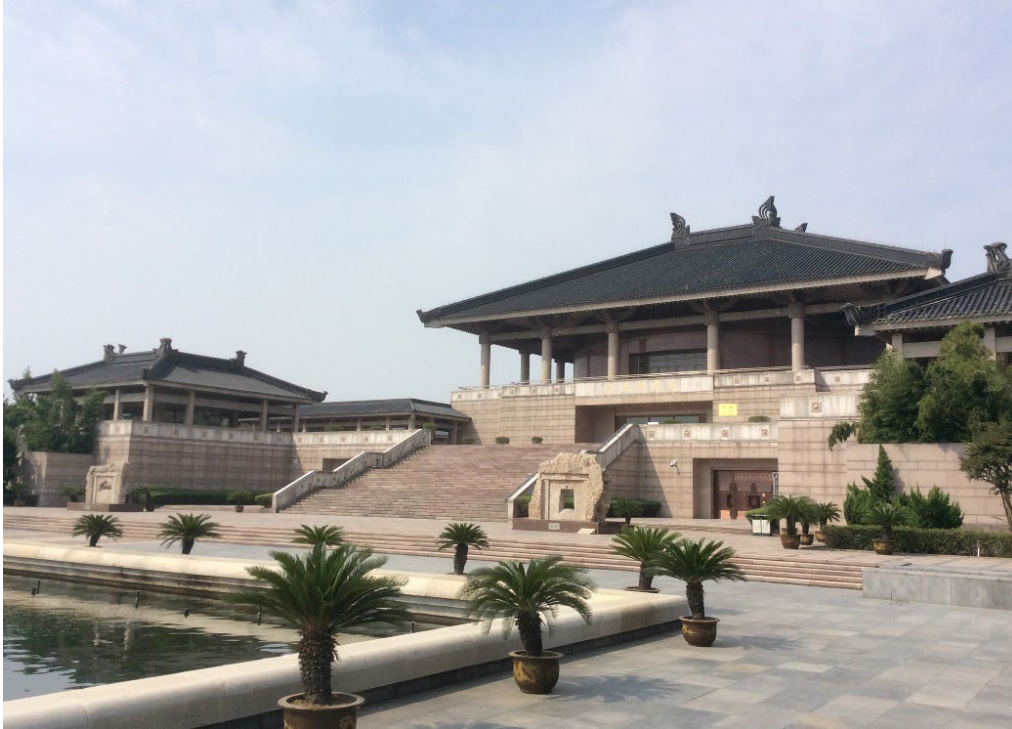
Figure 20. Main Building of the Confucius Research Institute, Qufu
