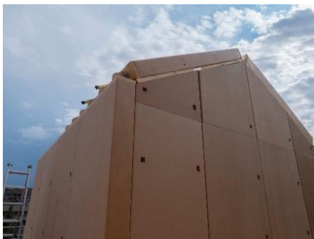
Figure 6. T-Box in Catania during the Construction
