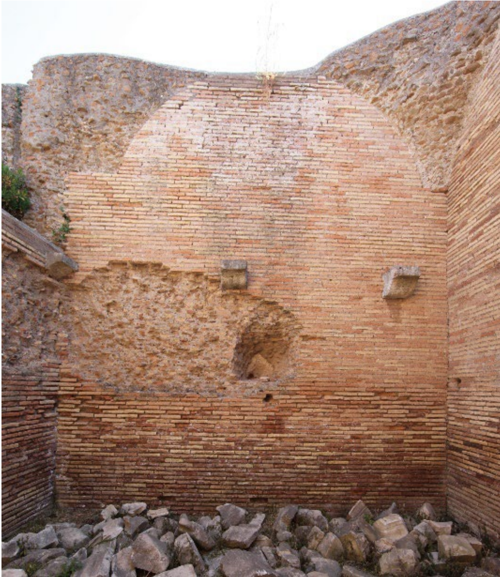
Figure 4. Outling Lunet Seen in Opus Testaceum
