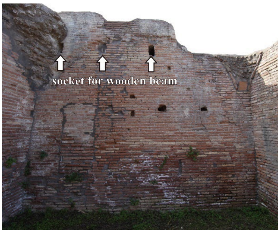
Figure 6. Conversion from Wooden-Beam-support to Cross-Vault-Support
