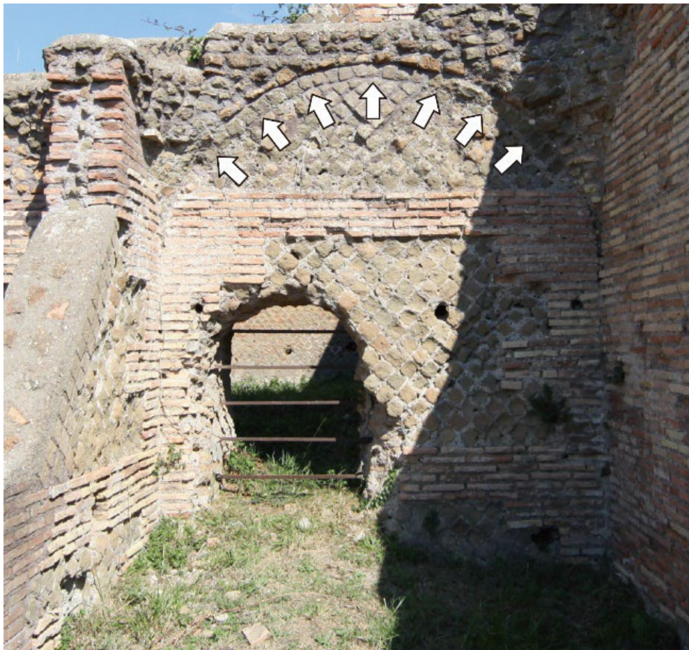
Figure 3. Outling Lunet Seen in Opus Reticulatum
