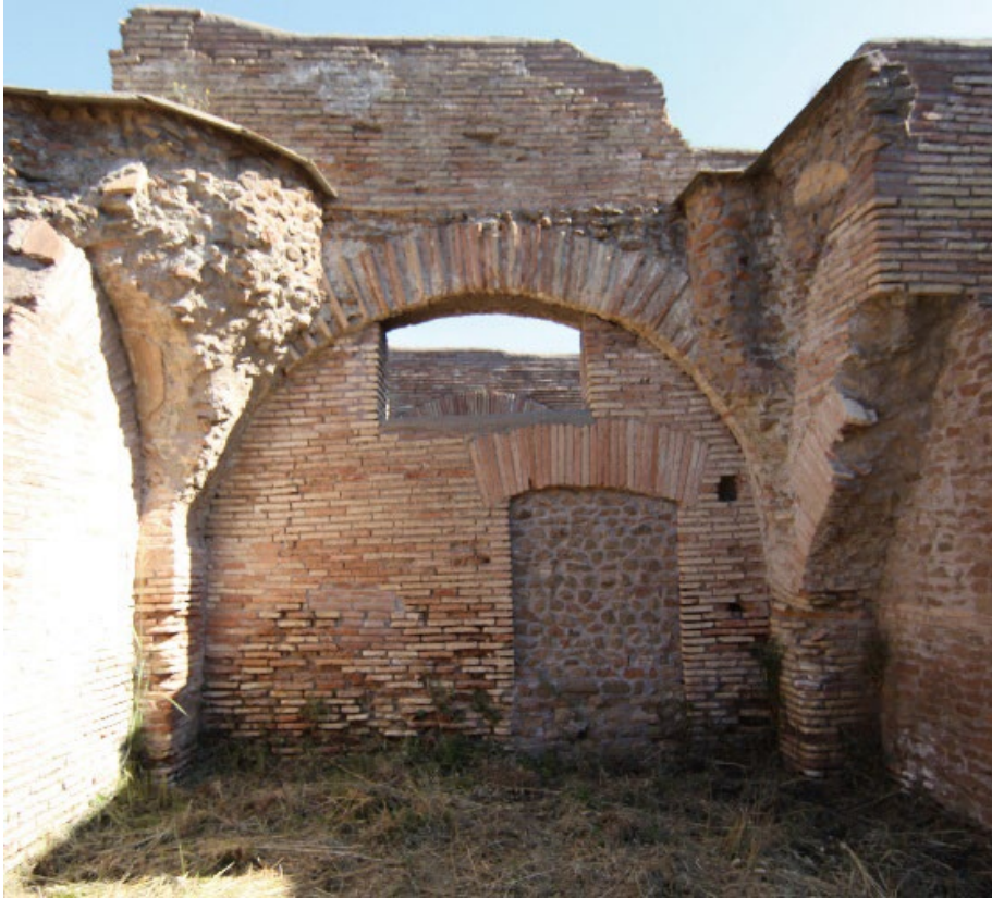
Figure 5. Building Partition Wall under Cross Vault
