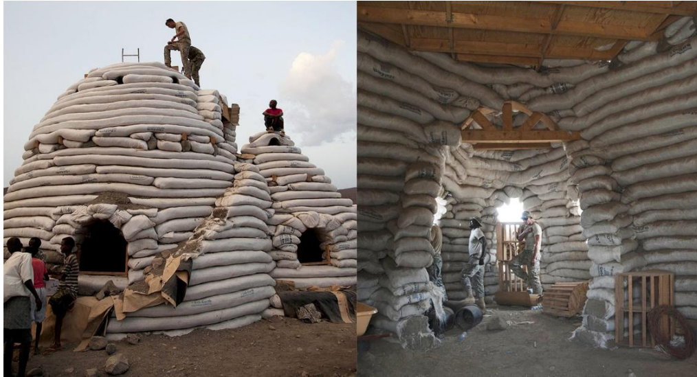
Figure 1. A Superadobe Structure Built in Djibouti (Africa) by Andrew Caya
