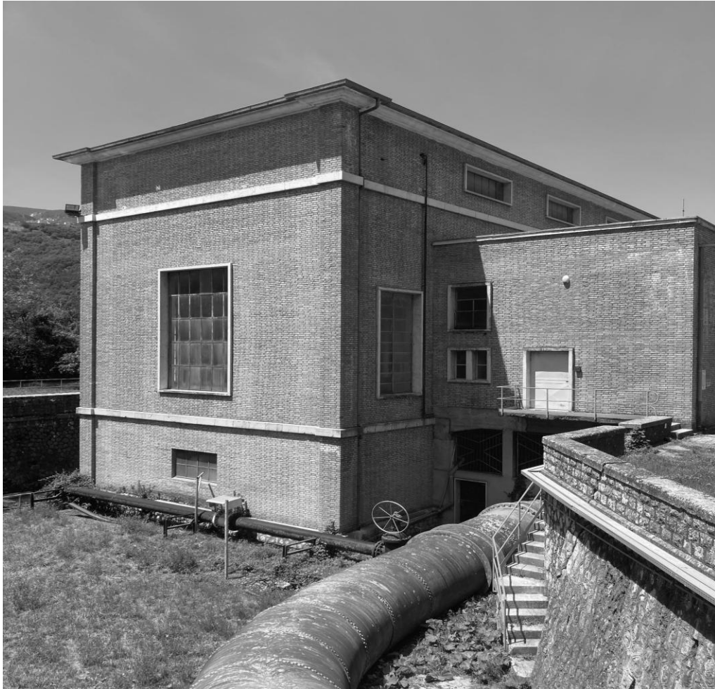
Figure 3. The “Torlonia” Plant in Canistro (Italy) and its Link with the Penstock (According to Fulvio Irace, the power plant is the central node of the hydropower system).
