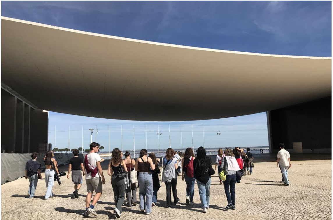
Figure 5. Álvaro Siza Vieira, Portuguese Pavilion. The Concrete Canopy (65×50 m span, 20 cm thick) is suspended in a Catenary Curve between Two Portal Frames Source: S. Rugins
