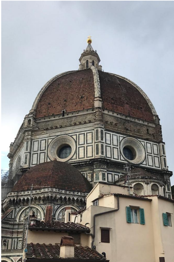
Figure 2. Filippo Brunelleschi, Dome of Santa Maria del Fiore, Florence (1420-1436) . The Brick Mass seems to rest with Impossible Lightness on the Octagonal Drum Source: S. Rugino
