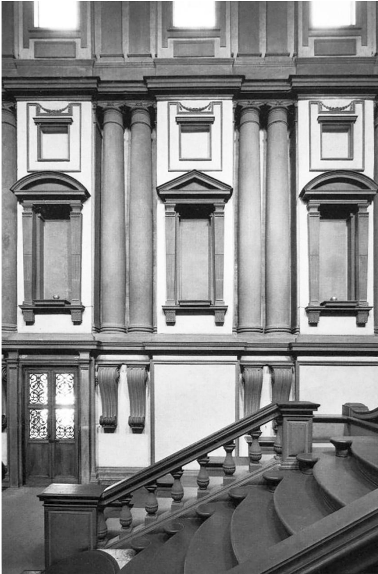
Figure 3. Michelangelo, Ricetto of the Laurentian Library, Florence (1524-1559). The engaged Columns Set within recessed Niches Reverse the conventional Hierarchical Relationship between Structural Support and Load Source: S. Rugino
