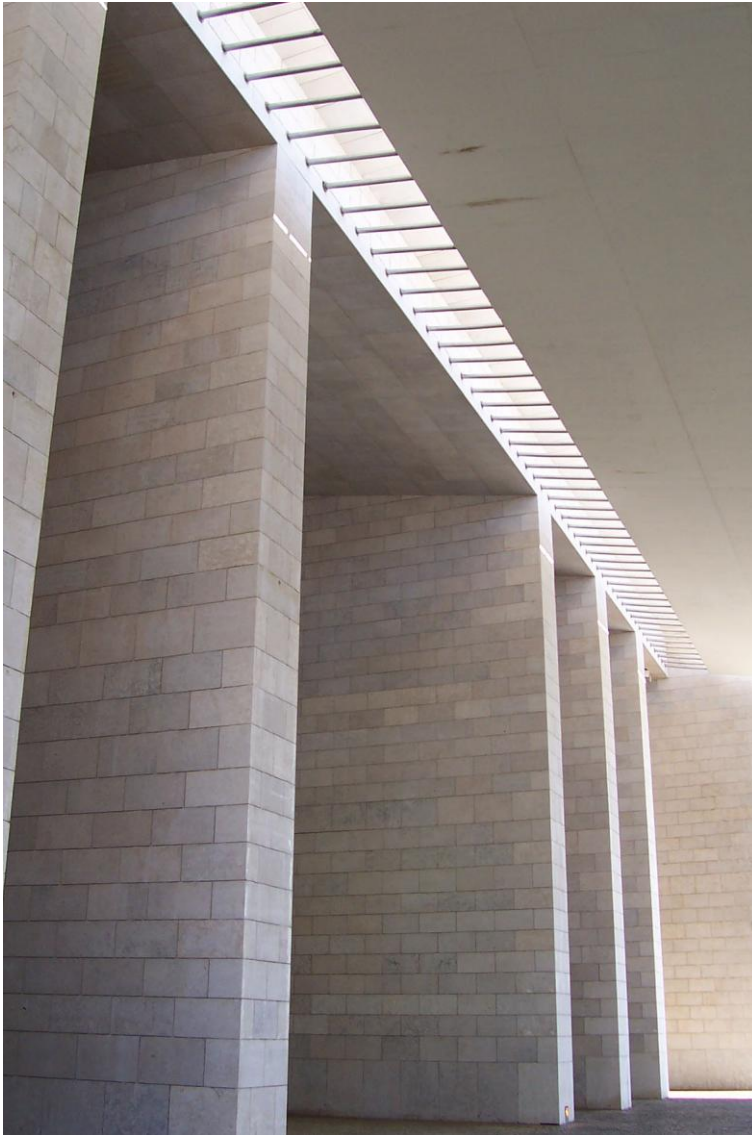
Figure 6. Portuguese Pavilion, Detail of the Roof-portico Junction. The 45° Bevel Optically Cuts the Structural Thickness, Accentuating the Perception of Structural Slenderness
