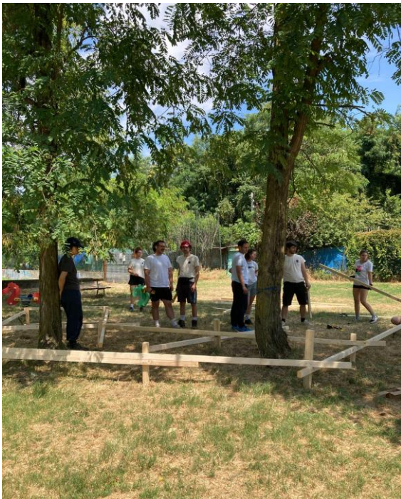
Figure 3. Building a Public Furniture around Trees, July 2025
