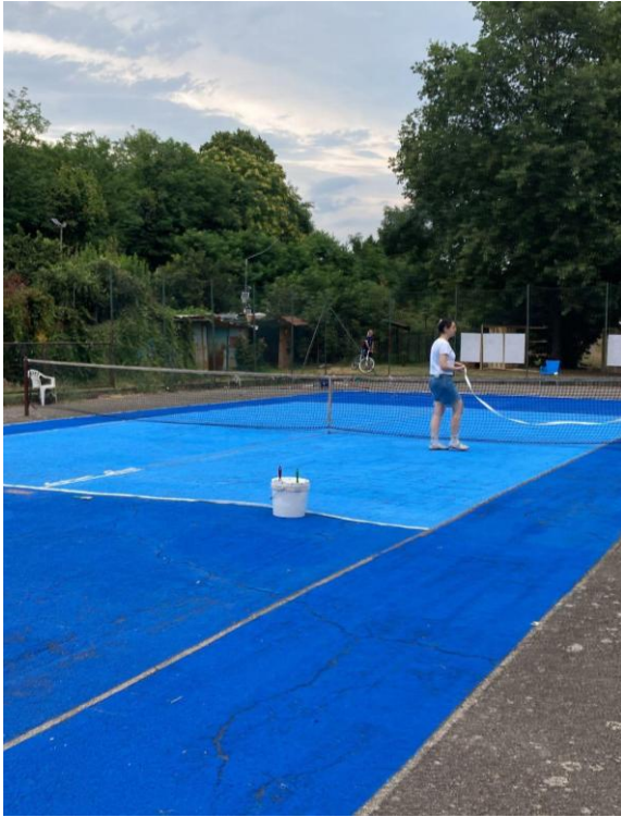
Figure 5. Repainting of the Tennis Court, July 2025
