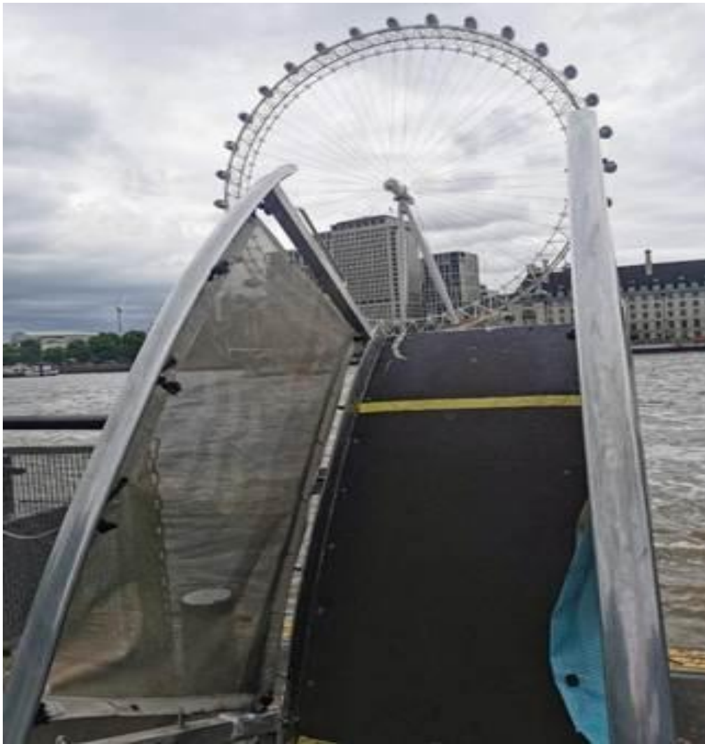
Figure 15. Ramp and Boarding Route Showing the Transition Between Pier and Vessel
