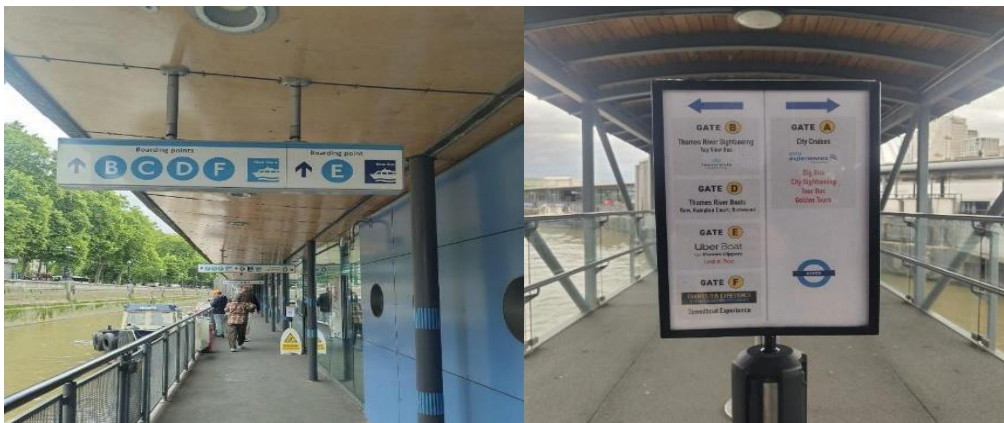
Figure 5. a., b. Westminster Pier, Division of the Piers
