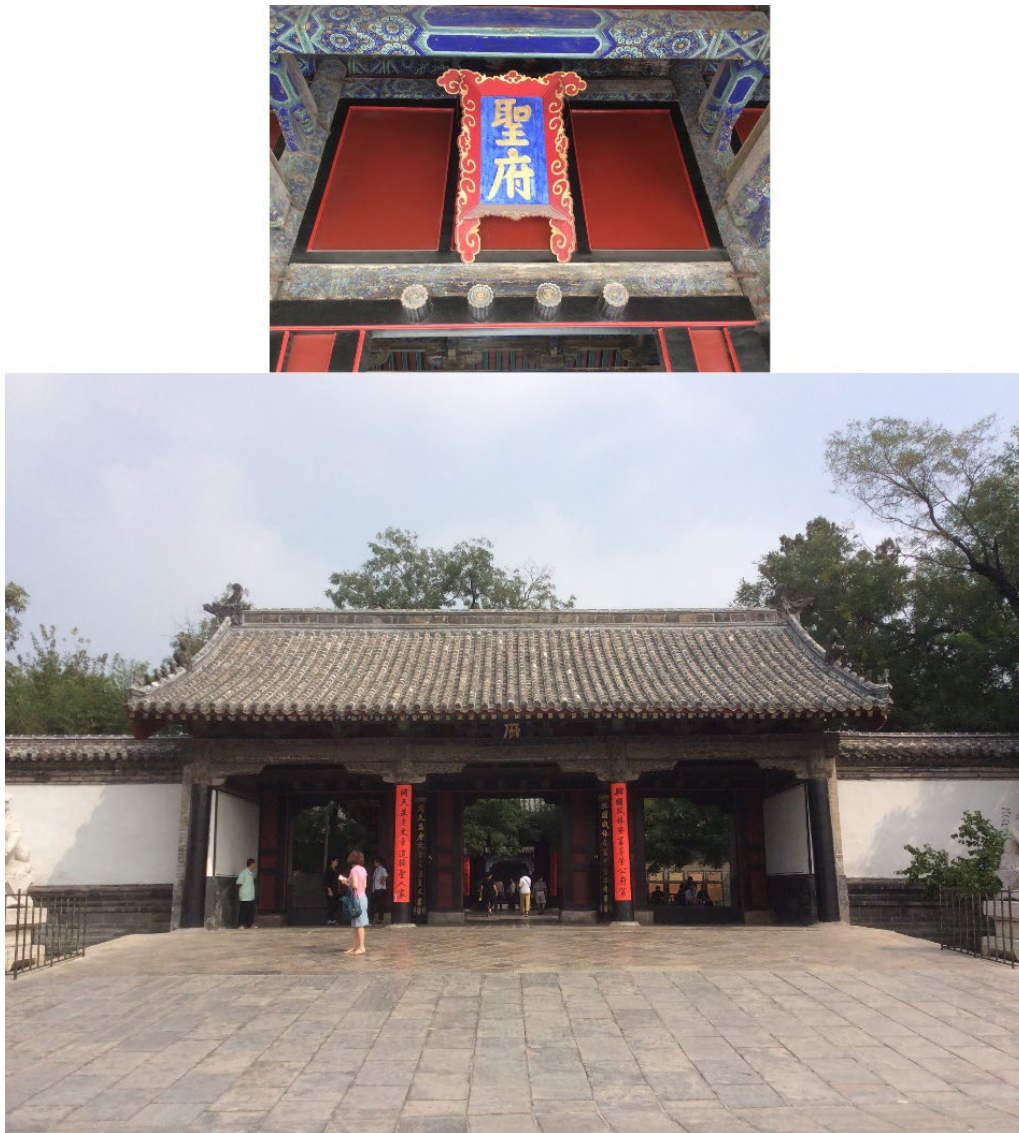
Figure 11. Main Gate of the Kong Family Mansion, Qufu Source: Photos by the author, 2017.
