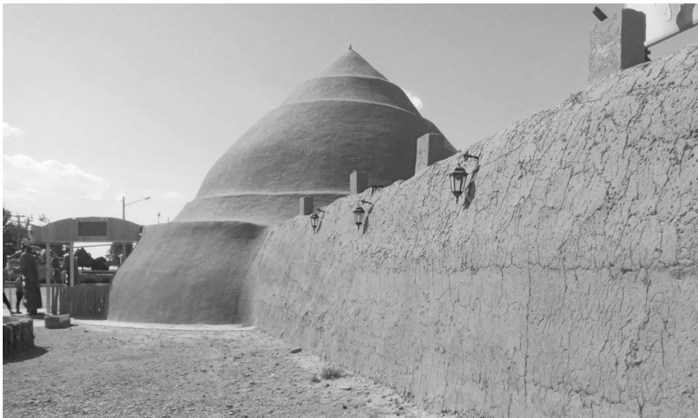
Figure 10. Yakhchāl of Kashmar Showing Icehouse and Shade Wall
