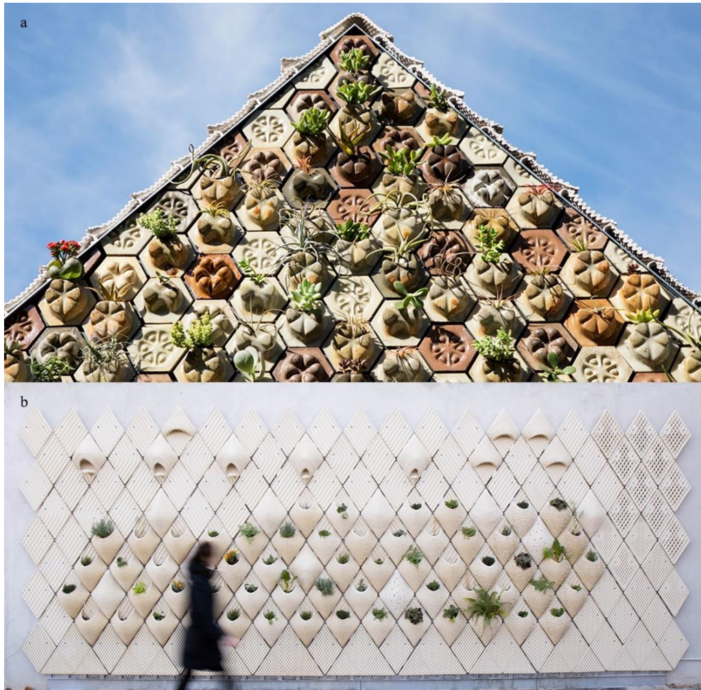
Figure 1. a) the 3D printed hexagonal tiles developed by Emerging Objects for the pavilion called Cabin of 3D Printed Curiosities ; b) CO-mida , designed and realised by the Advanced Architecture Group of the Institute for Advanced Architecture in Catalonia (IAAC)
