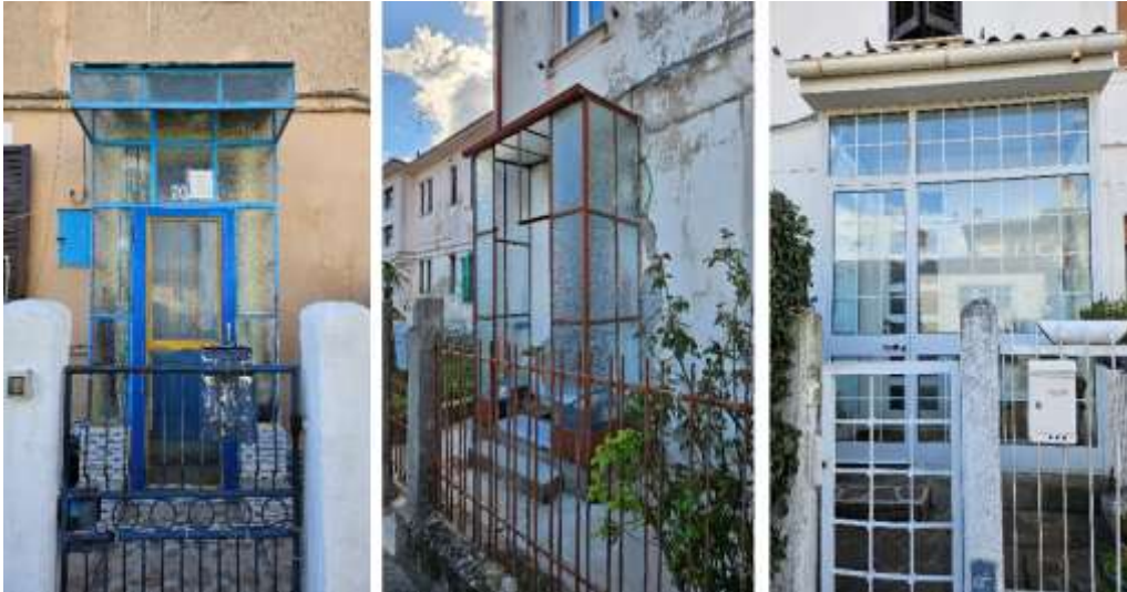
Figure 9. Existing Additions Providing Entrance Protection across Different Building Typologies in Panzano District: The Adopted Protective Systems Vary in both Type and Style
