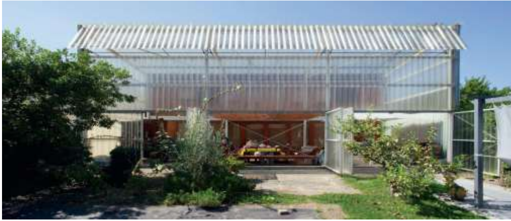
Figure 3. Lacaton & Vassal's Casa Latapie in Floirac (1993) (The Greenhouse is no longer subordinated to the building but becomes an equivalent architectural component that shapes the entire dwelling concept)
