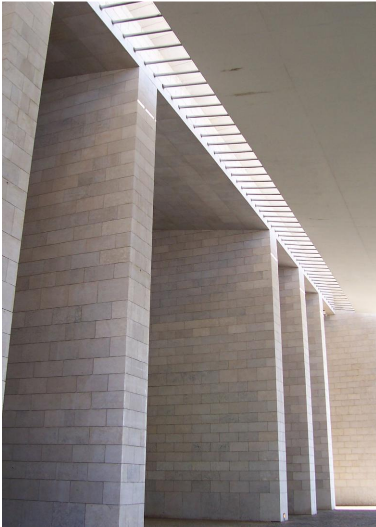
Figure 6. Portuguese Pavilion, Detail of the Roof-portico Junction. The 45° Bevel Optically Cuts the Structural Thickness, Accentuating the Perception of Structural Slenderness
