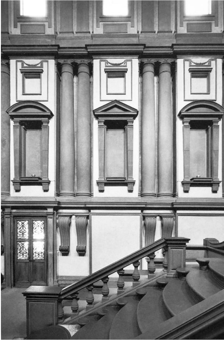
Figure 3. Michelangelo, Ricetto of the Laurentian Library, Florence (1524-1559). The engaged Columns Set within recessed Niches Reverse the conventional Hierarchical Relationship between Structural Support and Load
