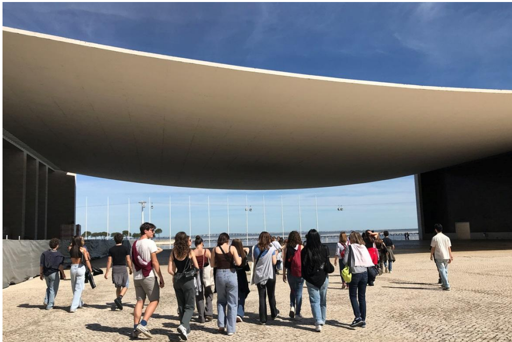
Figure 5. Álvaro Siza Vieira, Portuguese Pavilion. The Concrete Canopy ( 65 \times 50 m span, 20 cm thick) is suspended in a Catenary Curve between Two Portal Frames Source: S. Rugino.
