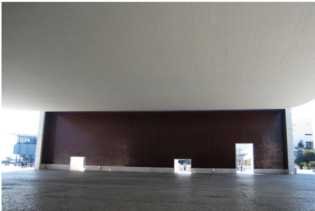
Figure 7. Portuguese Pavilion, underside of the Roof Structure. The Texture of the Maritime Pine (Pinus pinaster) Formwork combined with raking Light Produces a "Luminous Vibration" Phenomenon
