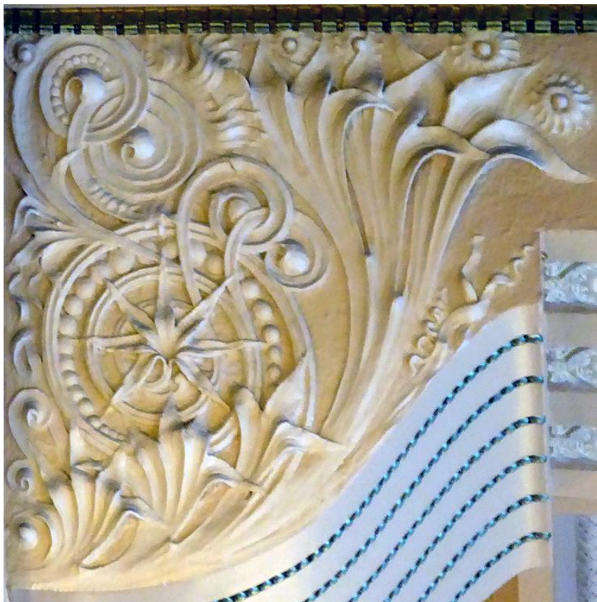
Figure 16. Beam Bracket Michigan Avenue Lobby
