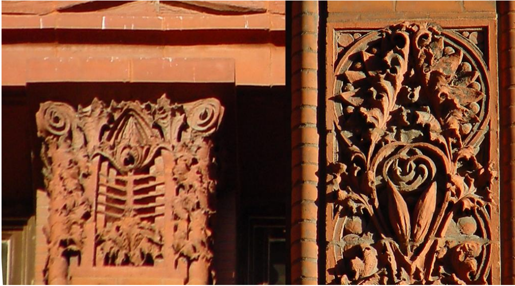
Figure 19. Wainwright Building Pier Capital (left) and Base (right)
