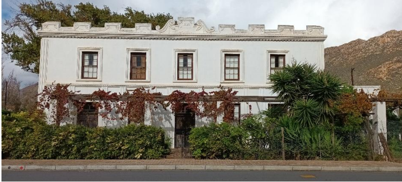
Figure 9. 40 Long Street, 1892; Cape Georgian House in Montagu. Photograph by author
