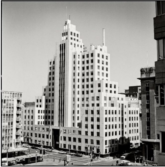
Figure 6. ESKOM House, Johannesburg (1934-1937). Original design by P. Rodgers-Cooke, completed by Pearse and Fassler. Photograph by Leon Krige 50
