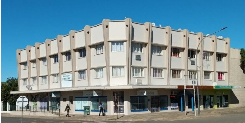
Figure 5.2. Caledon Court, 8 Church Street, Graaff-Reinet. Undated. Photograph by author
