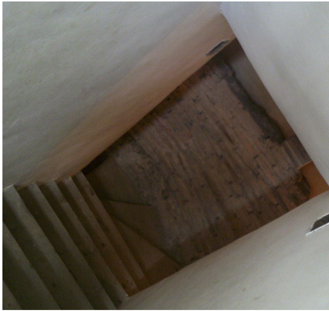
Figure 4 a, b, c, d, e. The Secret Fountain as it is Now (Nowadays one needs to go underground in order to access its water. That explains why today it is called 'the secret fountain'.)
