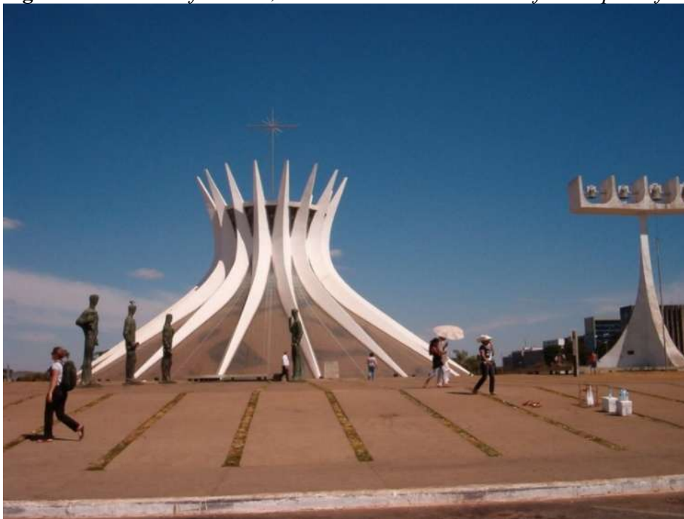
Figure 3. Cathedral of Brasilia, Located on the Central Axis of the Capital of Brazil
