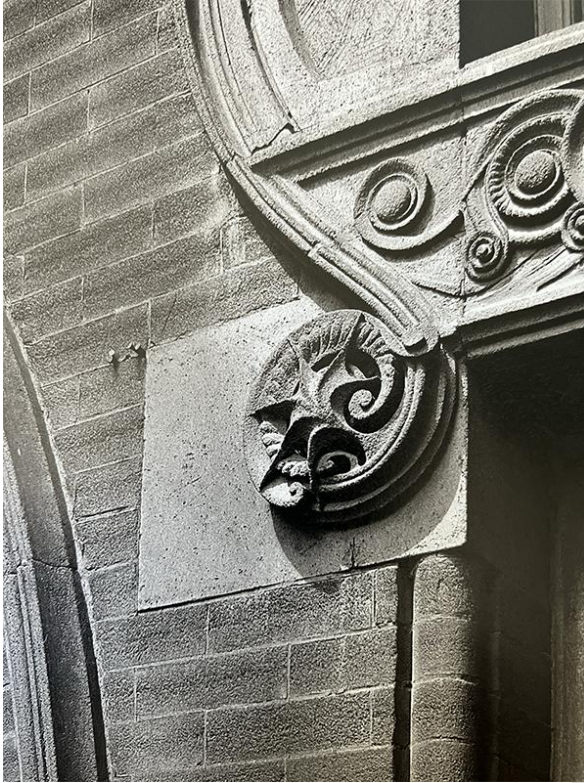
Figure 5. Ruben Rubel House Entry arch extrados efflorescence By permission of John Vinci
