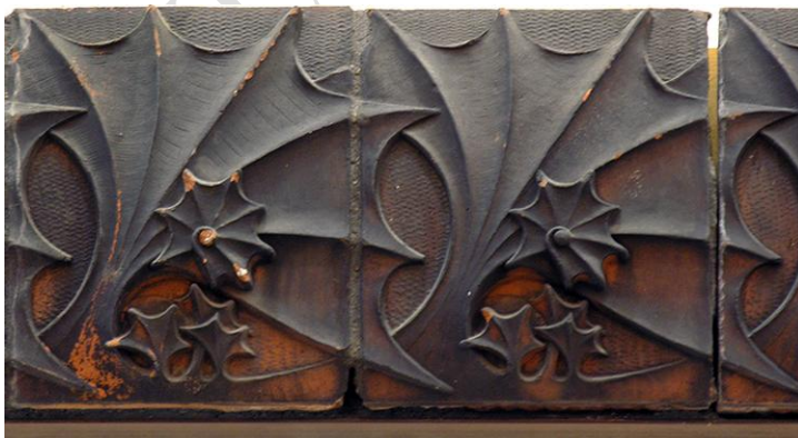
17 18 Figure 7. Lindauer House Stringcourse
