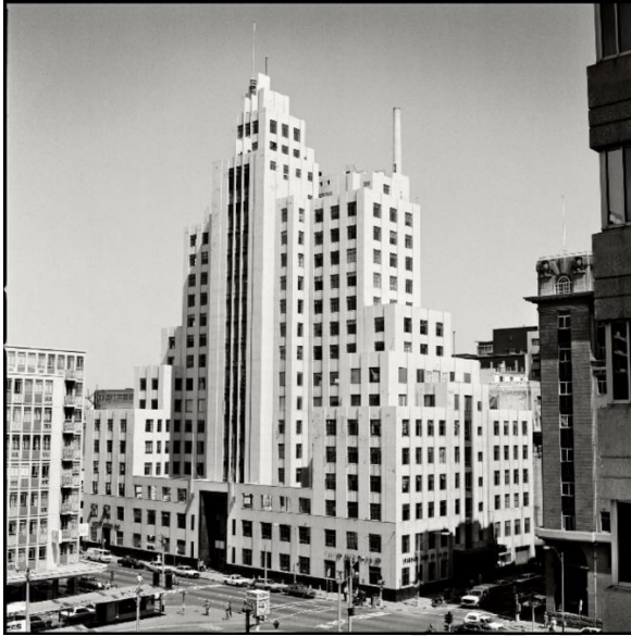
10 11 Figure 5. ESCOM House, Johannesburg (1934-1937). Original design by P. 12 Rogers-Cooke, completed by Pearse and Fassler 13 Photograph by Leon Krige 37
