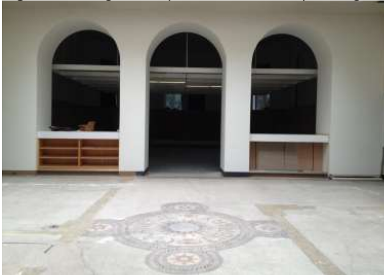
3 4 Figure 4. Carnegie Library Interior as Found by Koning Eizenberg
