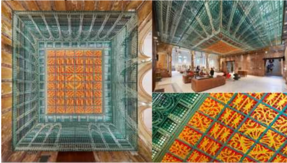
6 7 Figure 8. Ceiling Installation by FreelandBuck
