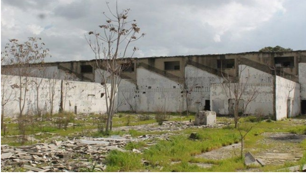
Figure 21. Current State of the Sümerbank Factory Site Showing Structural Decay and Abandonment
