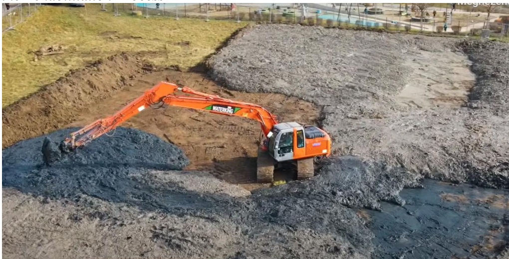
Figure 16. Ongoing Excavation and Drying of Sediment from the Lakes as Part of the Rehabilitation Process
