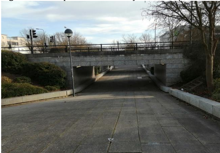
Figure 20. Underpasses in Milton Keynes in the Afternoon
