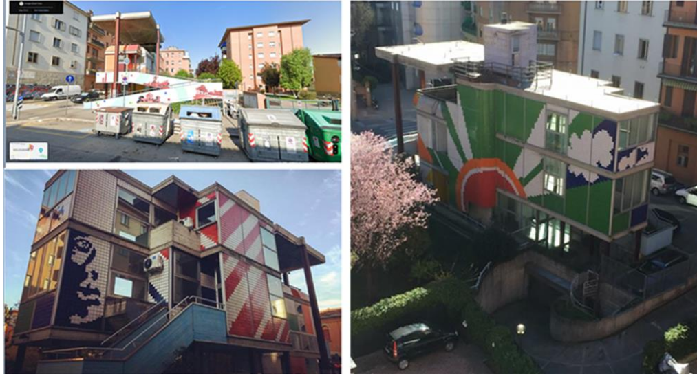
Figure 3. The Former Neighbourhood Library (Biblioteca Pelagalli), then Nursery School until 2012 – Current Headquarters of Hex, a Coworking Association, Privately Owned
